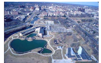
— Photo from Discovery Center Web Site
